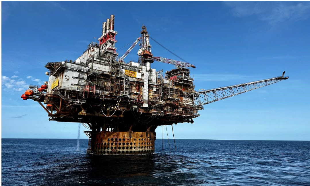
Figure 3-2 NCP Topsides (South Face)
