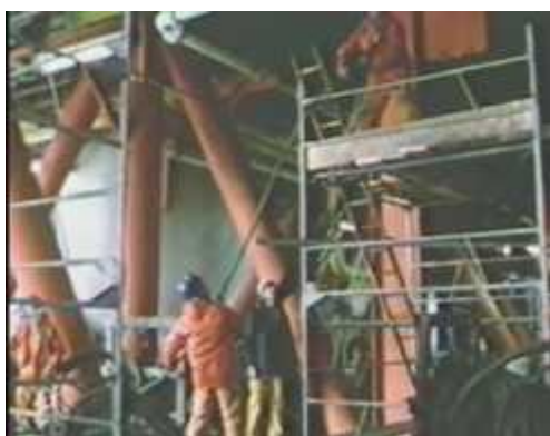
Figure 17: Hook Up and Commissioning of Modules
