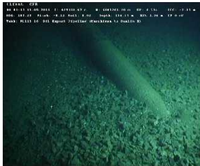
Figure 21: Transition exposed pipeline and rock profile
