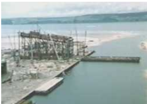
Figure 9: Jacket Prepared for Loadout
