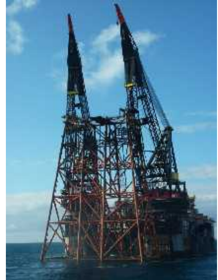
Figure 41: Jacket Removal Using a Heavy Lift Vessel
