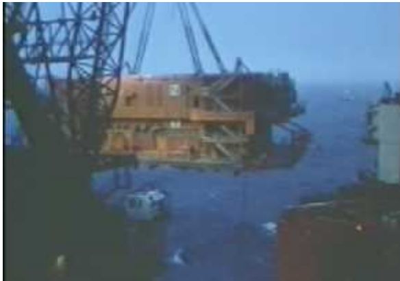
Figure 14: Installation of Topside Modules
