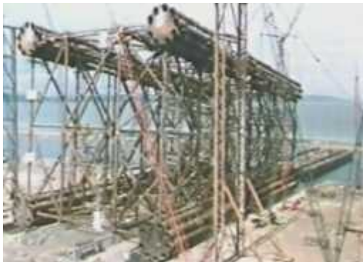
Figure 10: Loadout of the Murchison Jacket
