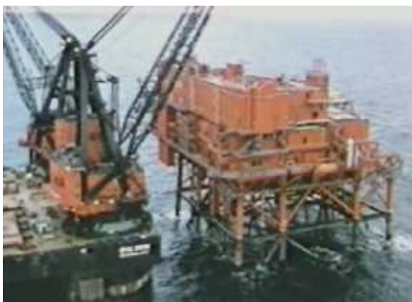
Figure 16: Second Level of Modules Being Installed
