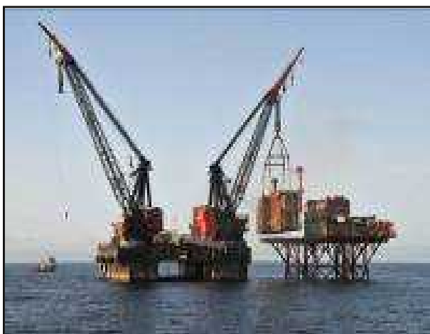
Figure 36: SSCV Lifts off Topside Module
