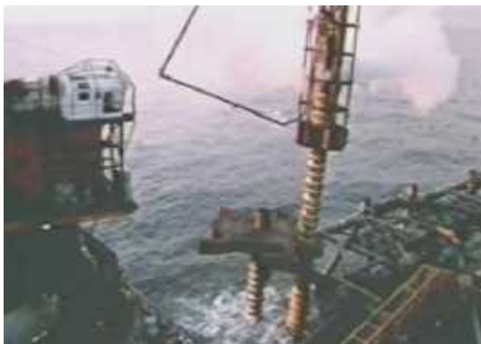
Figure 13: Jacket Piling
