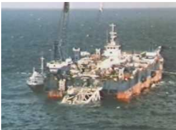
Figure 20: Laying the 16" OEL to Dunlin
